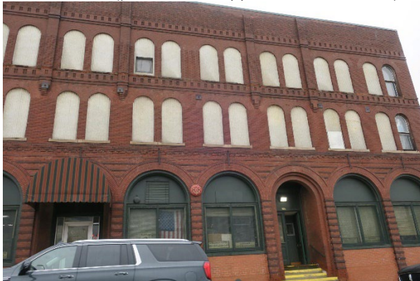
Downtown (potential for upper floor residential)
