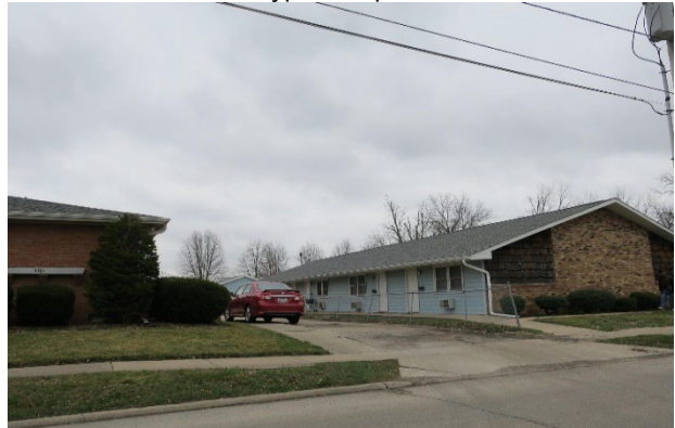
Typical multifamily (older stock)
