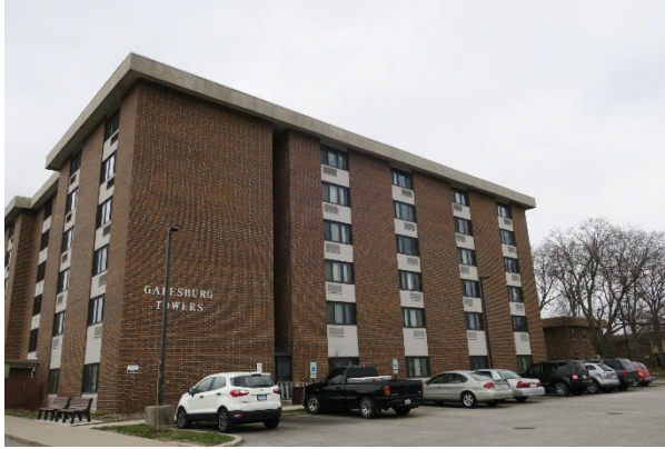
Typical higher density large (20+ units) multifamily
