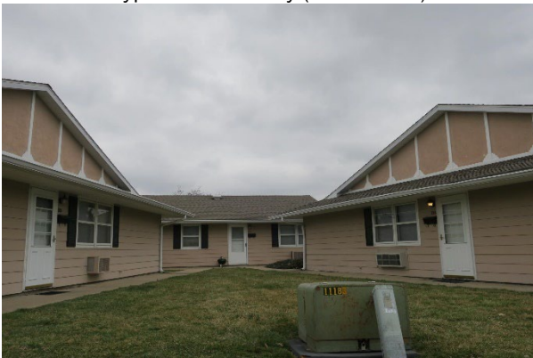
Typical multifamily (older stock)
