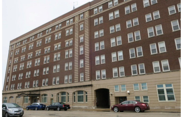
Typical higher density large (20+ units) multifamily
