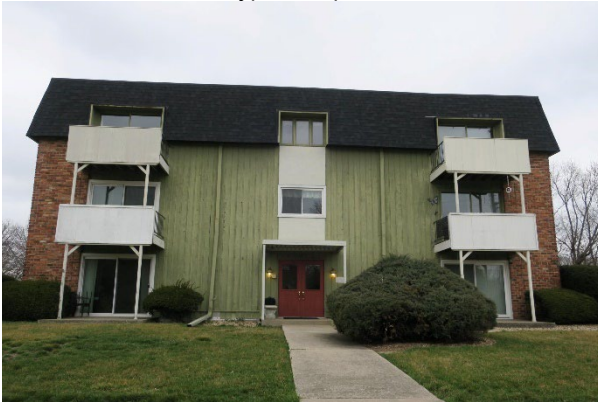
Typical multifamily (older stock)
