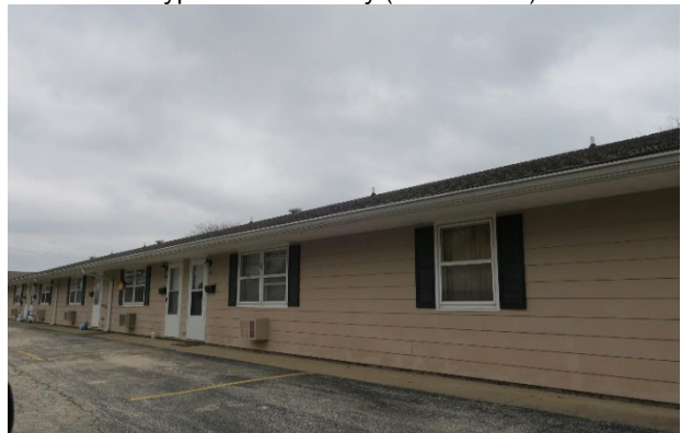
Typical multifamily (older stock)
