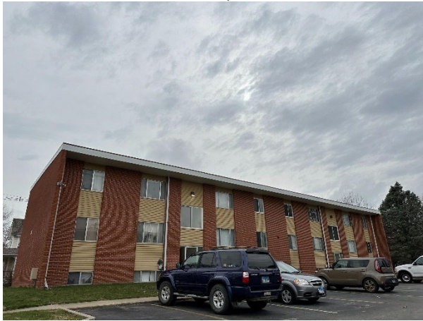
Knox Crest Apartments
