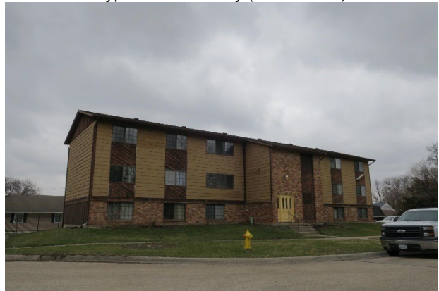
Typical multifamily (older stock)
